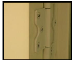
Hinge spacer installed.
