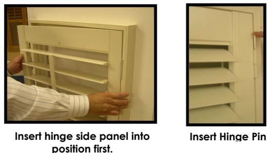
9. Once panel has been positioned and secured with the hinge pins, make sure shutter panel is even across the top and bottom. If panel is not even, shift (rack) your frame left to right until your reveal is even.
