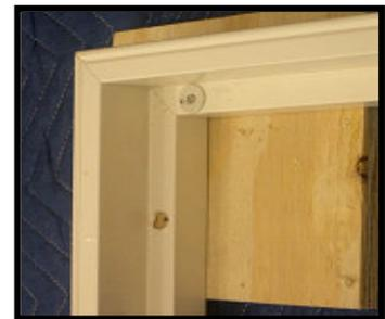
6. Position the assembled frame evenly around the window opening & secure with nail/screw (pre-drill) into the upper left frame ONLY. Shutter will be fully secured in later steps.
