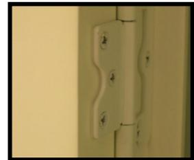
**Hinge spacer installed.**
