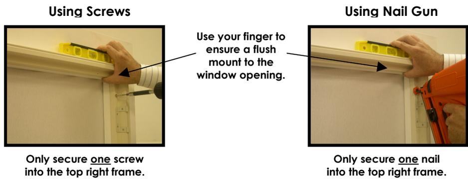
Once top right & left frame are secured, panel can be installed.
