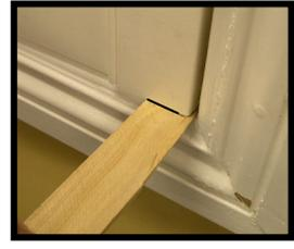
Push shim until stile is in line with shim mark.
