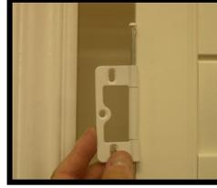
Completely install the hinge pin.
