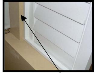
Finish by installing left light block.
