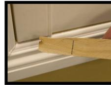
*Tip: The shim that is marked with a pencil, can be used as a guide for the right panel height spacing.*
